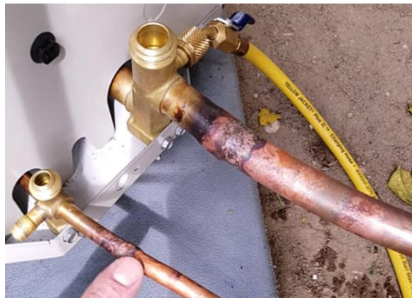
Fig. 6. Typical HVAC and refrigeration copper tube brazed joints during installation and assembly [49].
